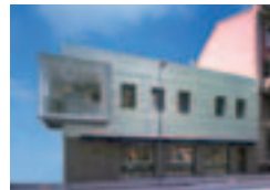
Japan Restaurant "My Sushi", Mailand, I Studio Clerici, Galizia e Totucci Associates, Arch. Lorenzo, Mailand Copermont S.r.l., Clusone (BG) TECU® Zinn
