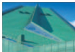
Urbis, Manchester, GB Ian Simpson Architects, Manchester Varla UK Ltd., Chester TECU® Patina
