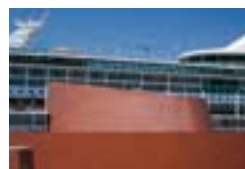
Harbour Terminal, Barcelona, E Grupo JG, Barcelona / BEA International, Miami (Florida), USA METAZINCO®, Madrid/Olloniego (Asturias) TECU® Classic
