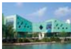
Yefei's Creative Street, Shanghai, VRC Alsop, London, GB; U/Jiang Architects & Engineers, Shanghai Hanchang Industrial Development Co., Shanghai TECU® Patina, TECU® Oxid, TECU® Bronze
