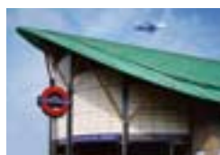
U-Bahn-Station Hounslow West, London, GB Michael Watkins (Partner), London, (Acanthus, Lawrence and Wrightson Architects) Broderick Structures Ltd., Woking TECU® Patina
